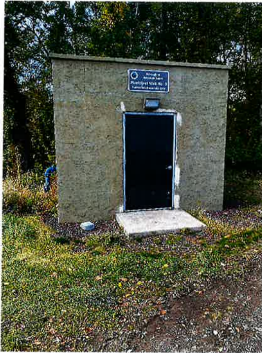
Figure 1: Well House No. 3
