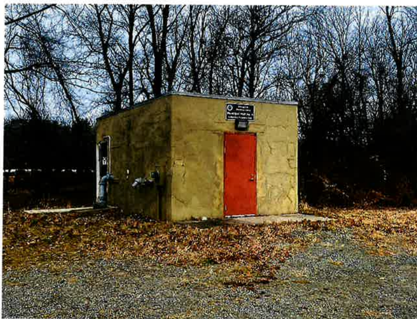
Figure 2: Well House No. 4
