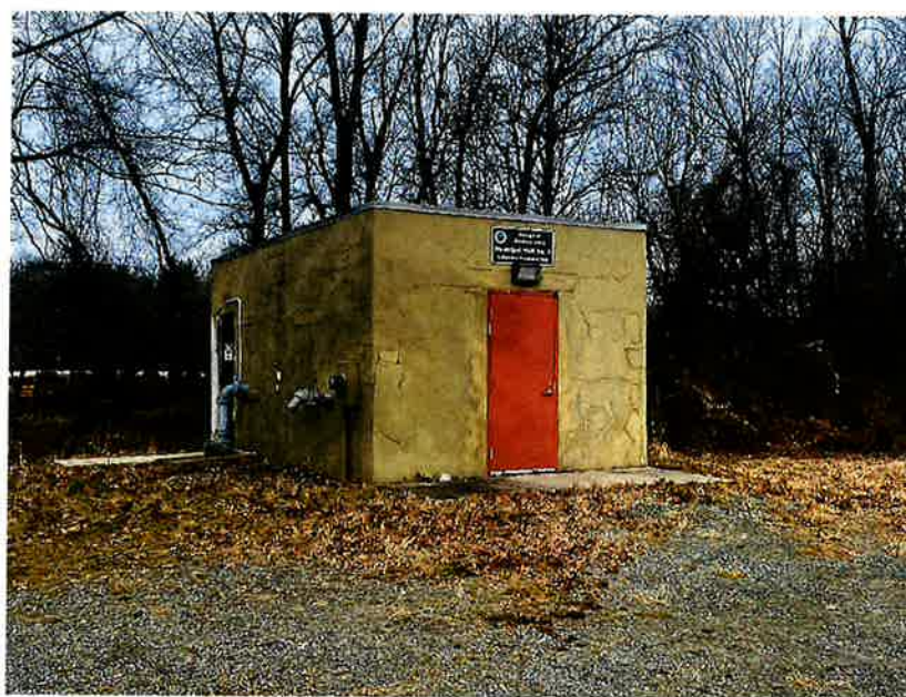
Figure 2: Well House No. 4
