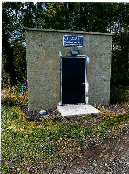
Figure 1: Well House No. 3
