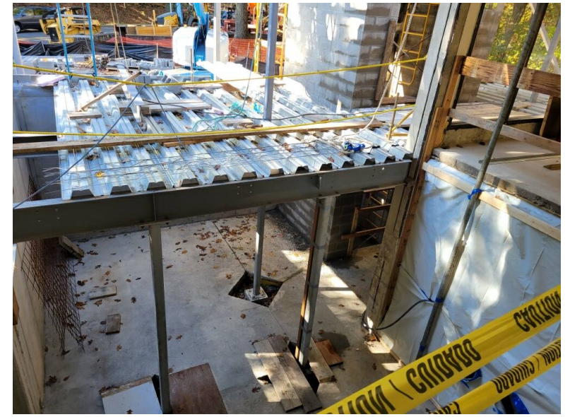
Steel Supports and Decking at Front Addition
