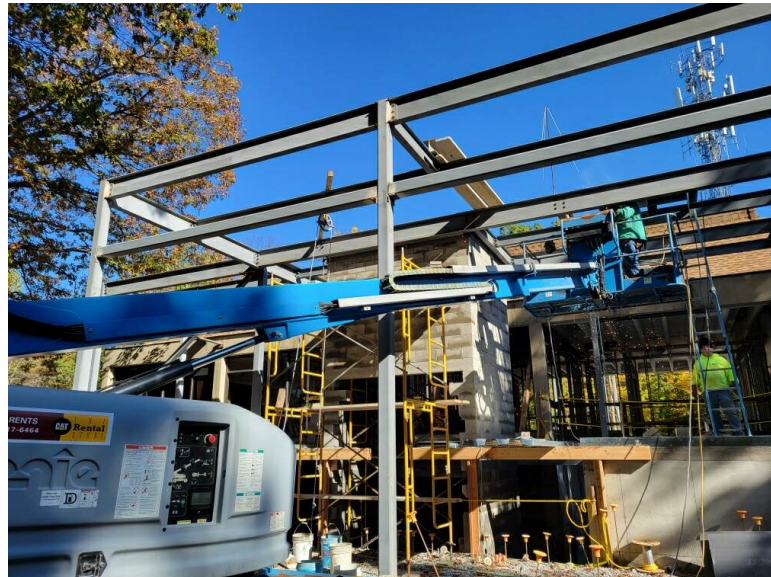
Front Addition Steel and Elevator Shaft Block
