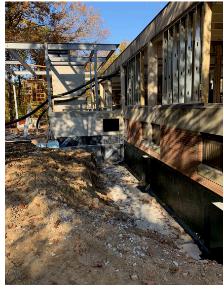
New Waterproofing Along Existing Building
