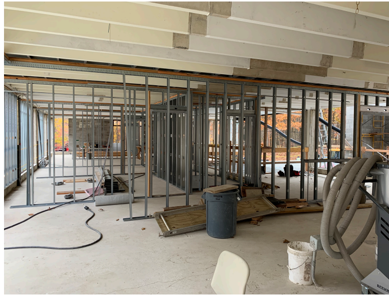
Upper-Level Interior Framing In Progress
