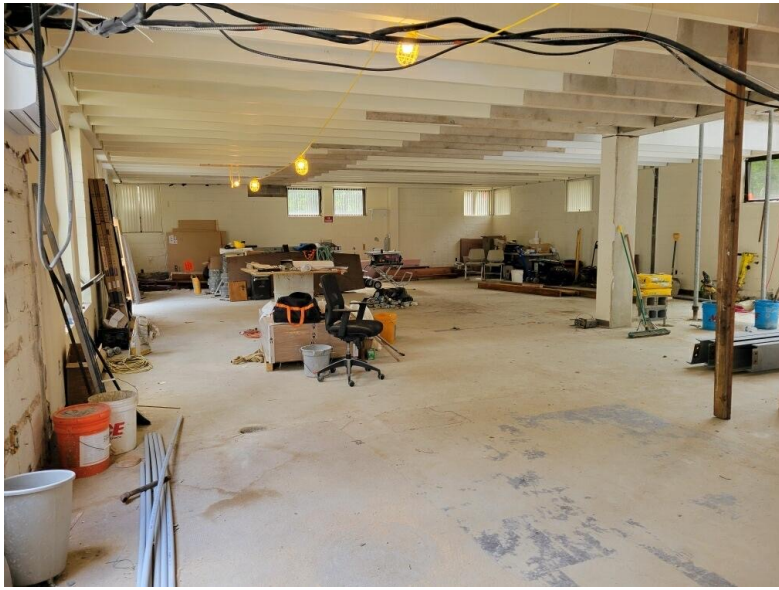
Lower-Level Demolition Completed
